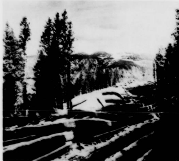
WORKING AHEAD OF THE CREWS, timber is cleared away and salvaged by Dave Menauy of Red Lodge. He cuts the timber along the road path, removes and burns all slash, and will use the timber for milling purposes. —(Enterprise photos)
